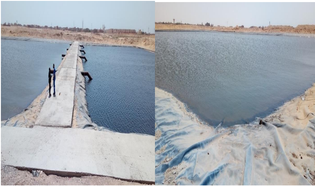
Fig.(12): Typical lined evaporation pits for evaporating produced water
