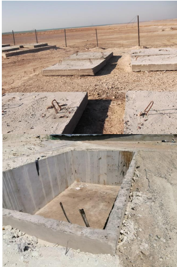
Fig.(17): Typical underground temporary storage (concrete bunkers)
